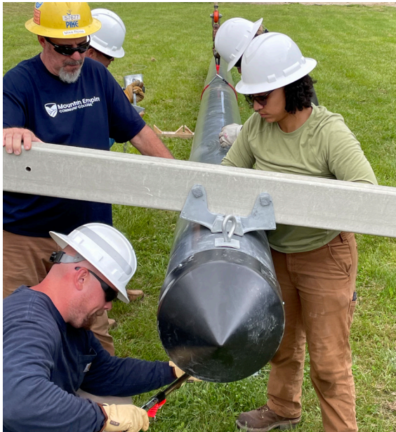
FIG. 8.1 Crossarm structural connection
